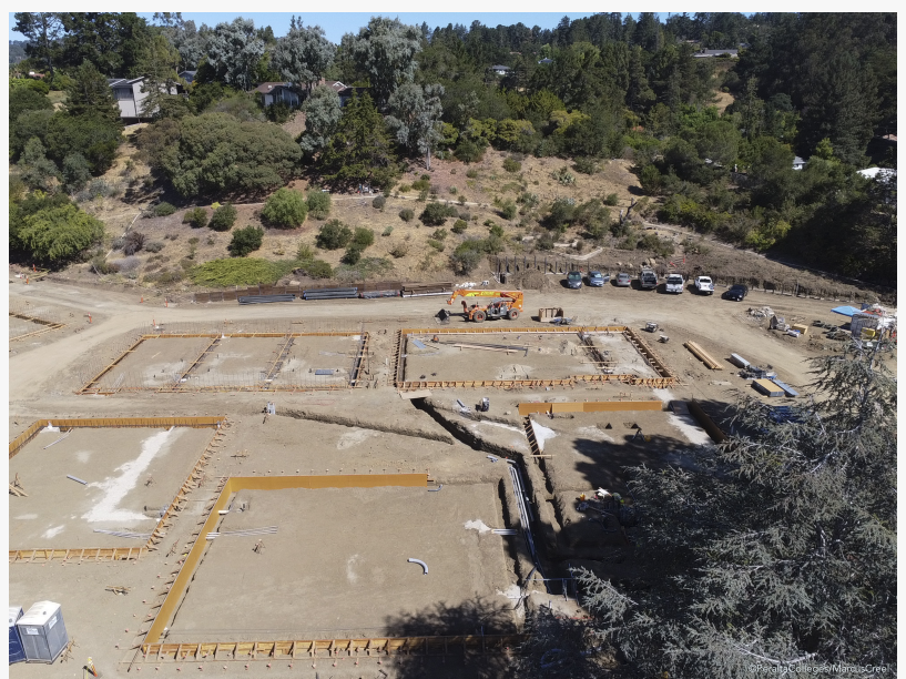
Merritt College Horticulture Complex Project - Photo Credit: The Peralta Community College District - Marcus Creel
