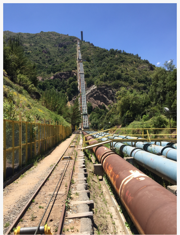
Seismic Rehabilitation in a Remote Location 2
