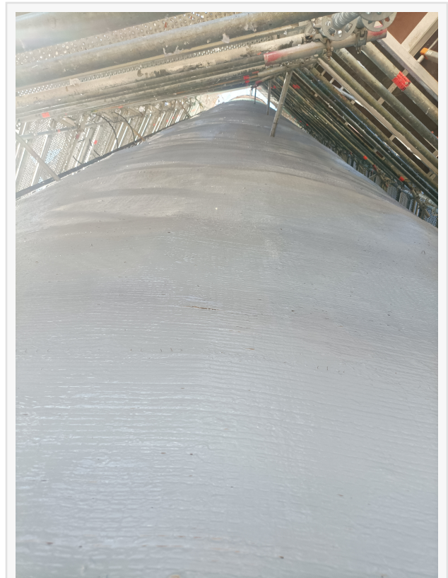
Seismic Rehabilitation in a Remote Location 3
