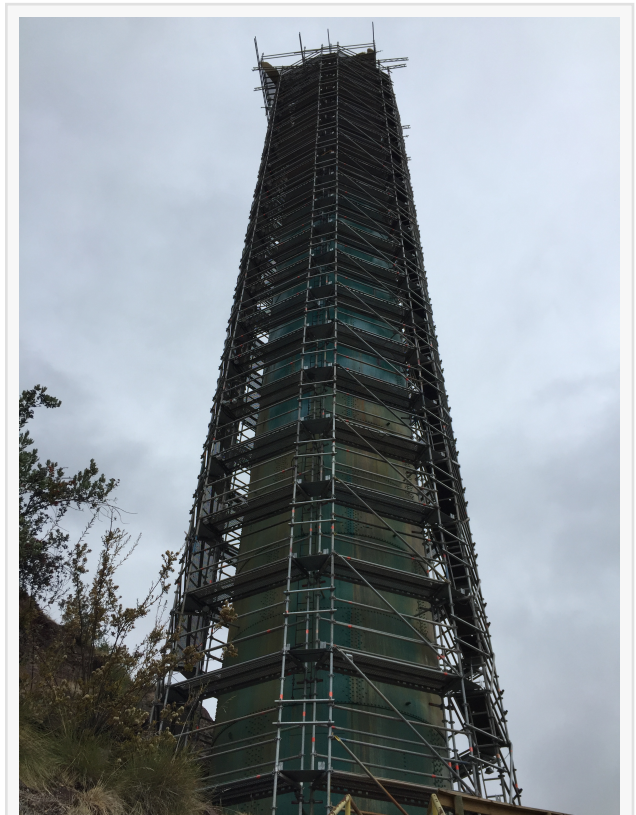
Seismic Rehabilitation in a Remote Location
