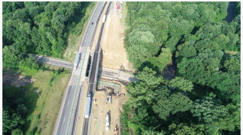
Acrow - Temporary Bridge, Michigan
