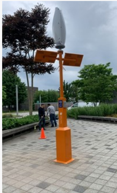
ZW Charging Station in Tilburg
