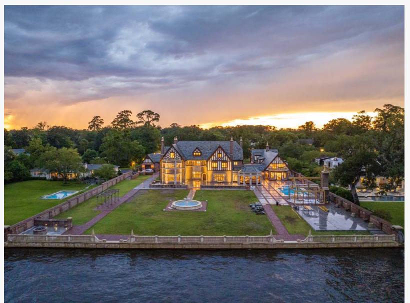
3730 Richmond Street | Jacksonville, FL
