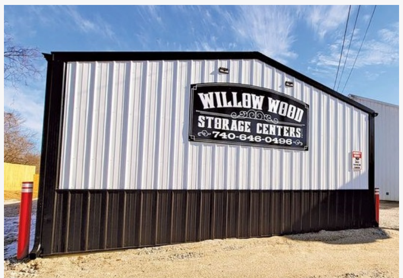
Willow Wood Storage Centers
