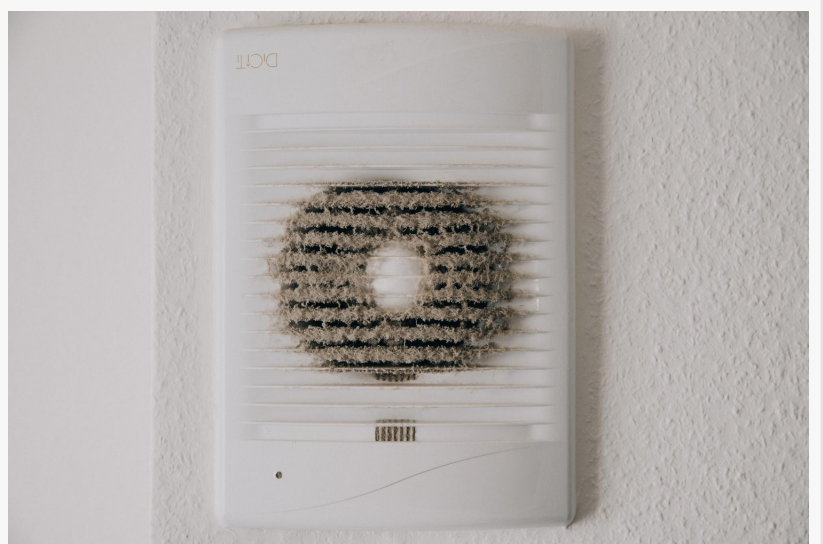
Air Duct Cleaning Services
