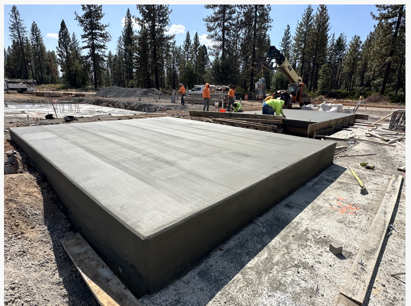
More foundation work at Hat Creek Bioenergy Facility (Burney, Calif.)
