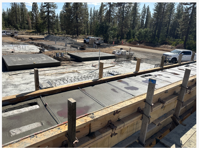
Foundation work at Hat Creek Bioenergy Facility (Burney, Calif.)
