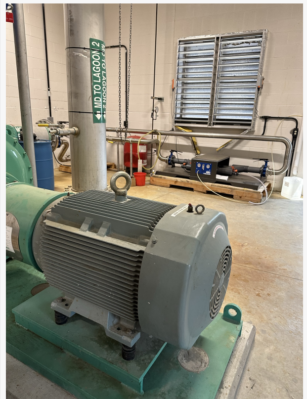
Moleaer Nanobubble Generator Installed at Meister Plant
