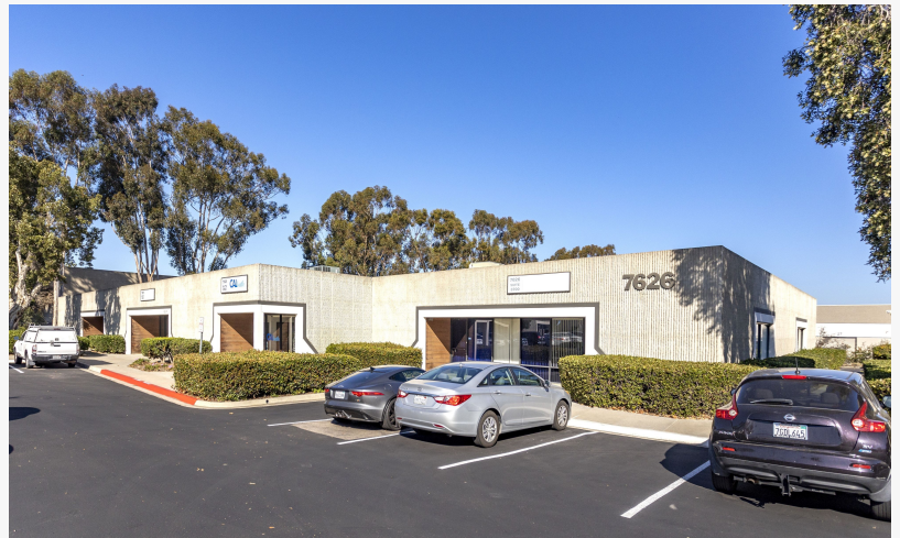
7626 Miramar Road - Miramar Business Park
