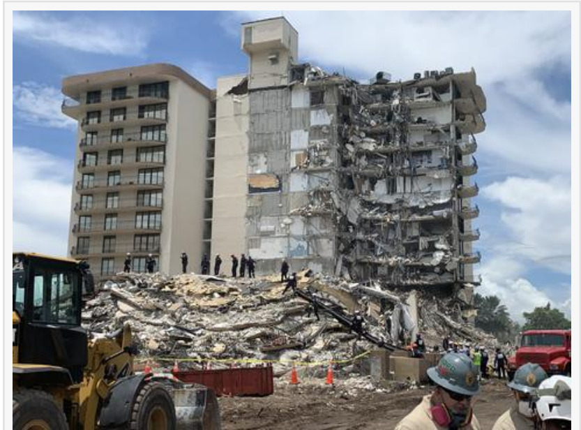
The site of the partially collapsed Champlain Towers South in Surfside, Florida. Image courtesy of NIST.
