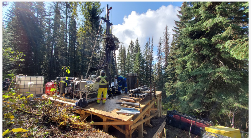
Image 1: Sonic Infrastructure Geotechnical Drilling Underway Within WSF Area
