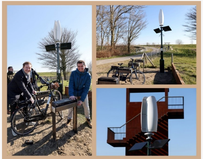
ZW Charging Station in Nissewaard
