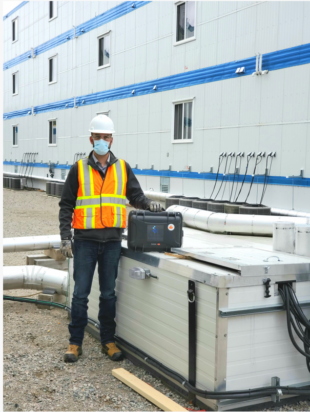
Sampling at Remote Sanitary Wastewater Lift Station
