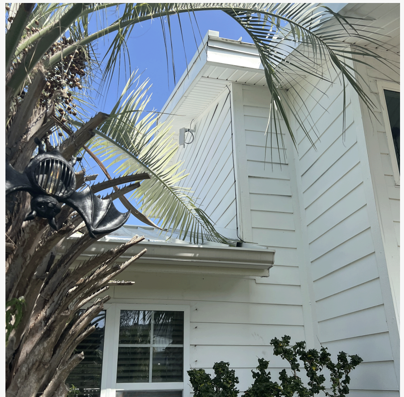
Installation of GigaBlu receiver at customer's home.
