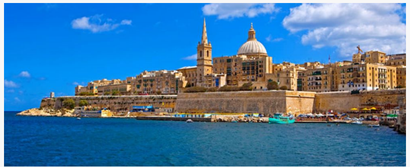
The Valletta Skyline before restoration works began
