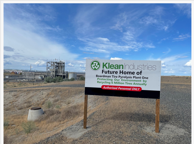
Klean Industries Boardman's end-of-life tire recycling & recovered carbon black site.
