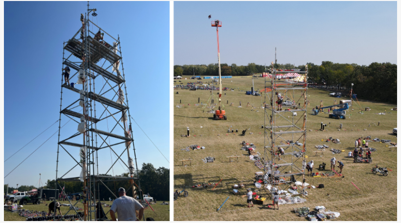
The 39-foot scaffolding adorned with pyrotechnics was a prominent feature on the Sky Wars field and in Scott Smith's winning display. Photos by Sam Christensen.
