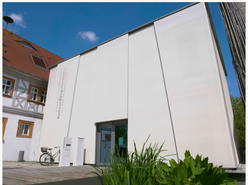
Administration building with a roho textile facade for passive building air conditioning.
