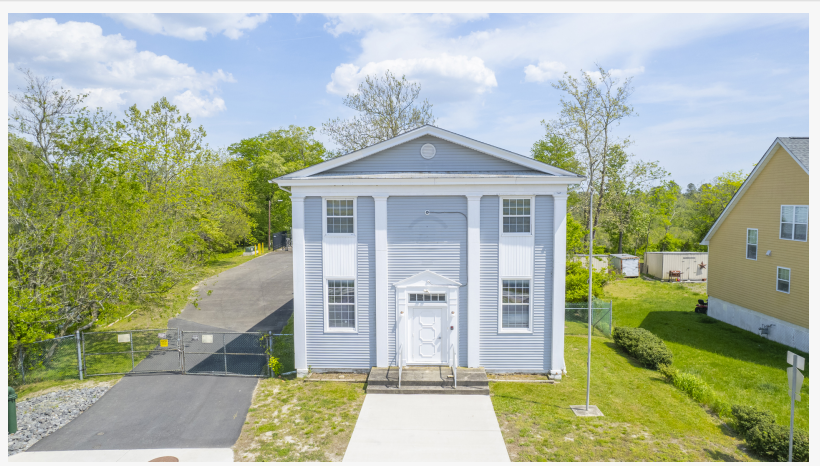
Former Masonic Lodge
