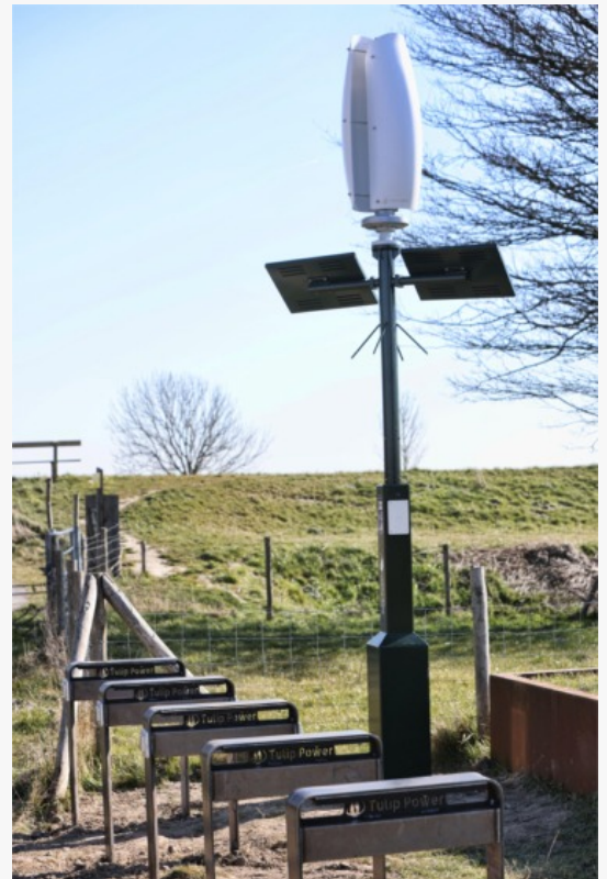
Flower Turbines Charging Pole at Nissewaard
