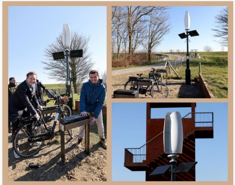
ZW Charging Station in Nissewaard
