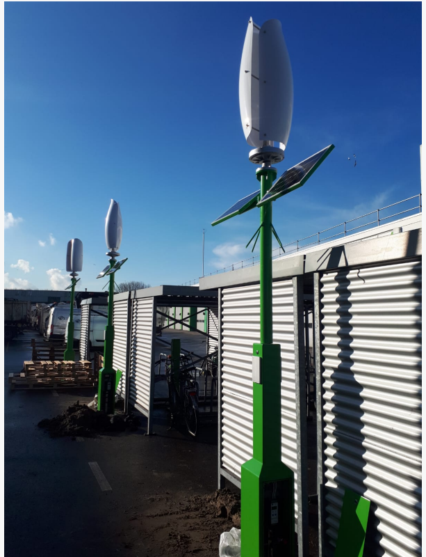
Wind and Solar E-bike Charging Poles
