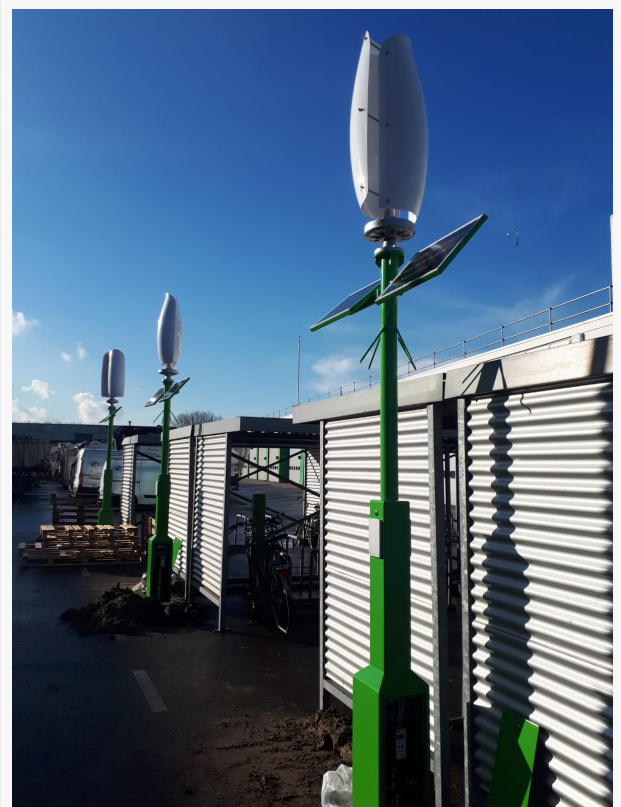
Wind and Solar E-bike Charging Poles
