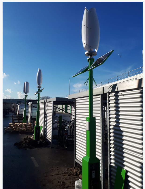
Wind and Solar E-bike Charging Poles
