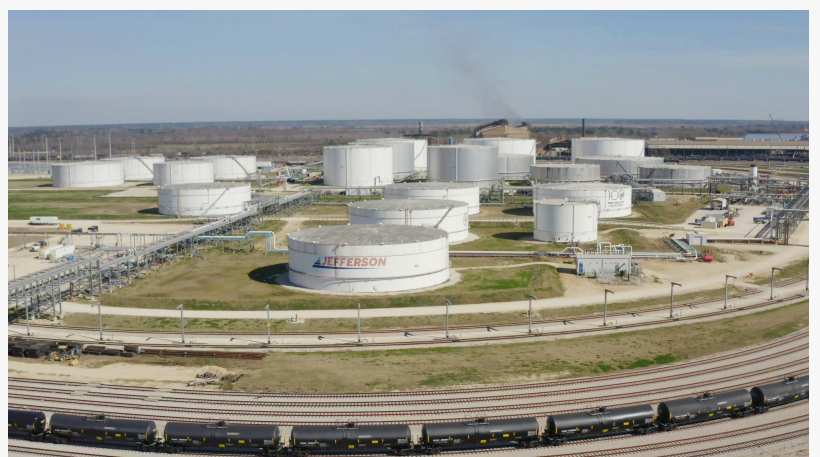
Jefferson Energy Project
