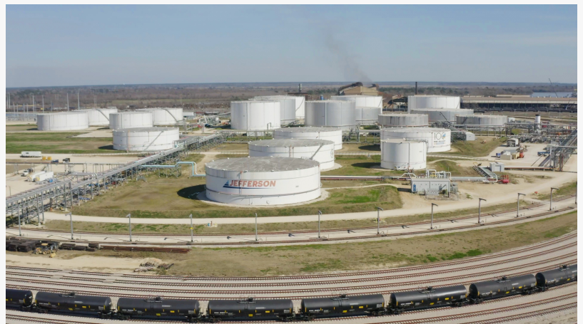
Jefferson Energy Project
