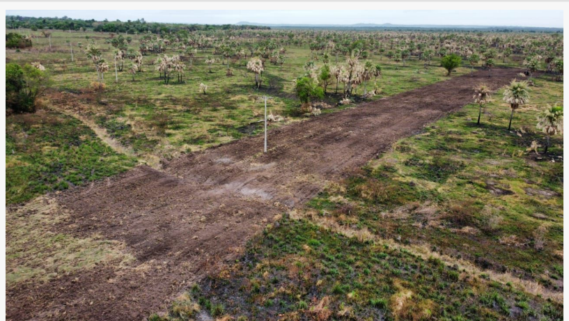
Construction work has begun on the Aldera Resort.
