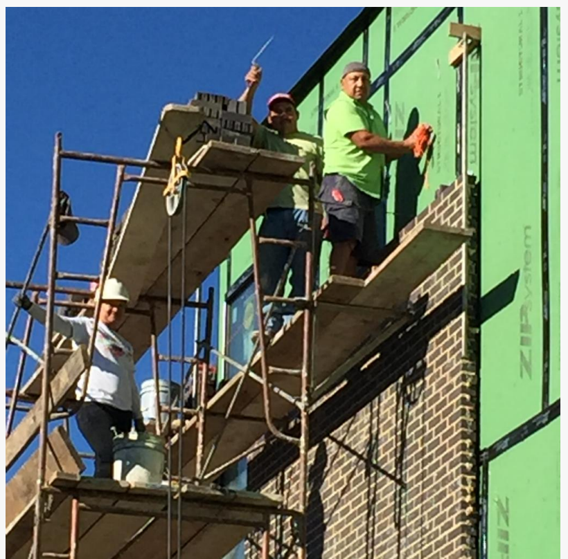
masonry work in dallas
