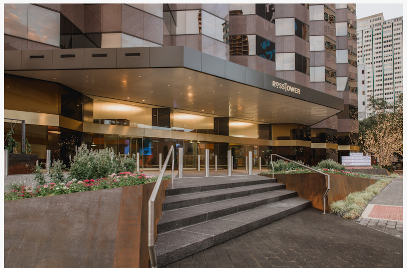
Front of Building New Barbieri Law Firm Location
