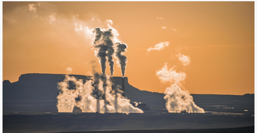
Cold winter power restrictions in the UK Energy generation in desert areas
