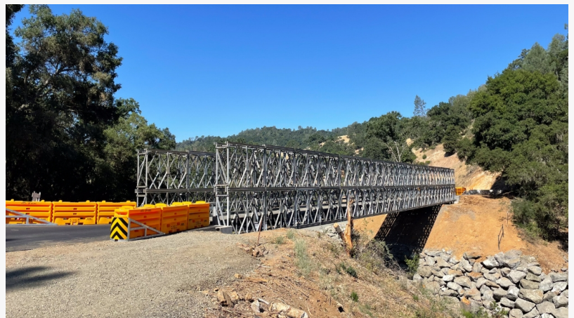
Acrow Bridge - San Luis Obispo County, California
