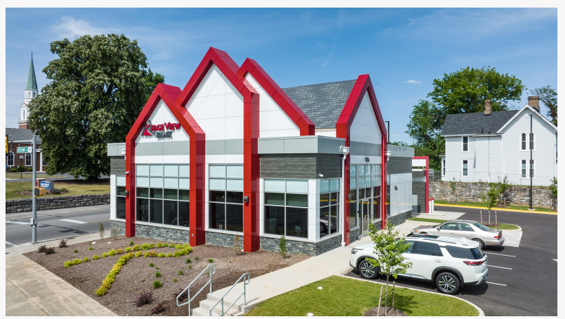
Ridgeview Bank Salem by G&H Contracting and Thompson Masonry - Meagan Williams Photography
