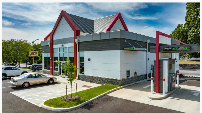
Ridgeview Bank Salem by G&H Contracting and Thompson Masonry- Meagan Williams Photography
