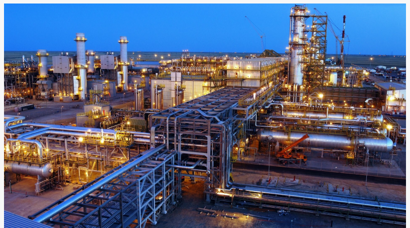
Oilfield Chemicals Market
