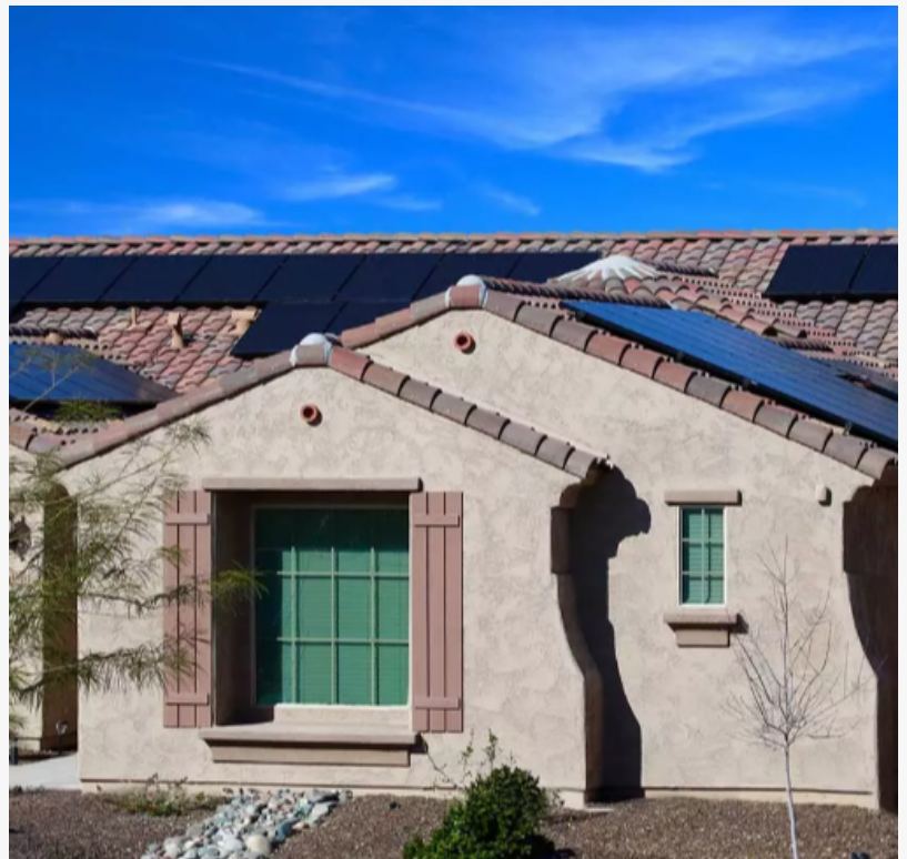
Sunsolar Solar System Installation
