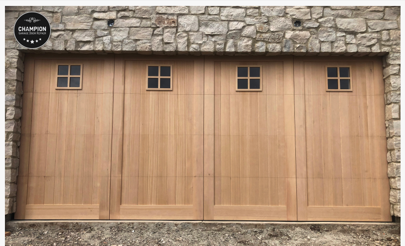
Custom Garage Door Installation in Huntington Beach
