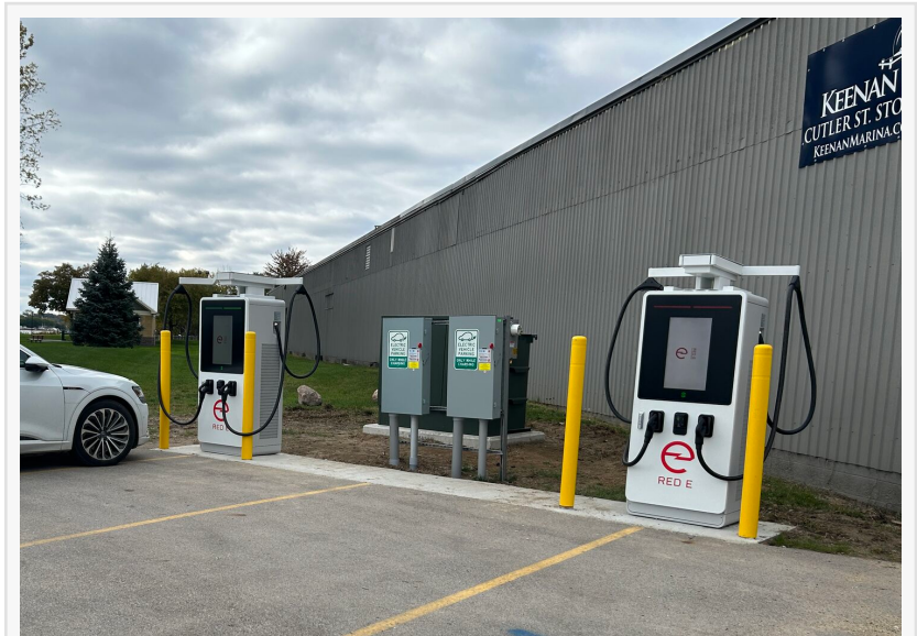
Two Dual-Port DC Fast Charging Stations in the Village of Spring Lake
