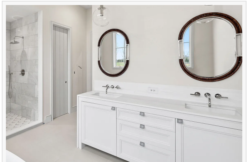
Hide-A-Trim Bathroom Counter Installation
