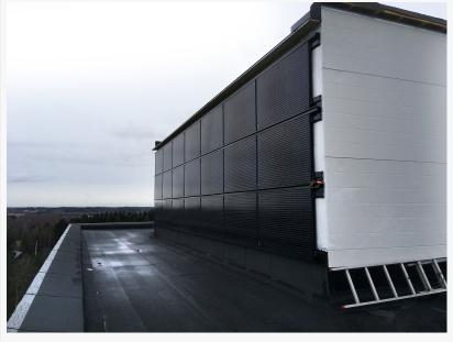
them – and it doesn't require physical effort from the technician either. The material is Scandinavian steel, which can be painted according to the customer's preferences. The parts are commonly delivered with a sleek black finish, which gives the entire setup an impressively stylish look.
