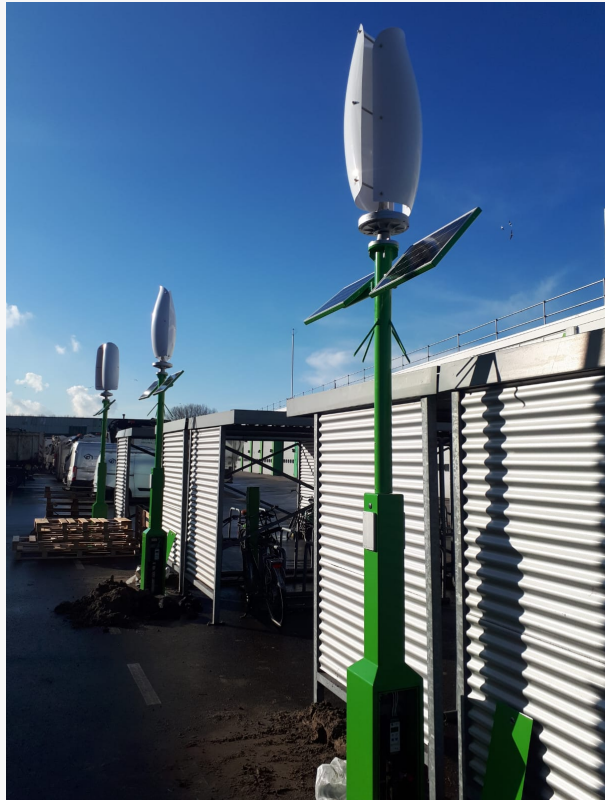
Wind and Solar E-bike Charging Poles
