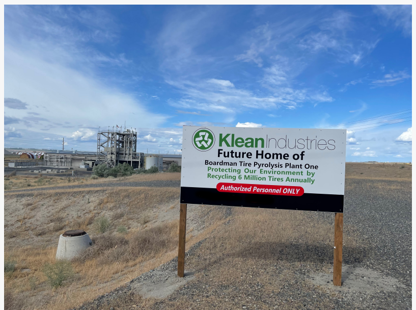
Klean Boardman end-of-life tire recycling & recovered carbon black site.
