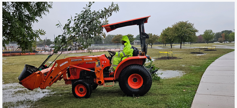
The City of Dallas Park & Recreation department helps prep the site for planting, pre-drilling the holes, and more.
