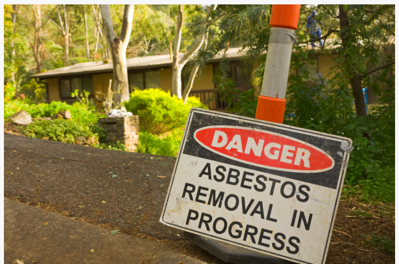
Australian house undergoing asbestos removal
