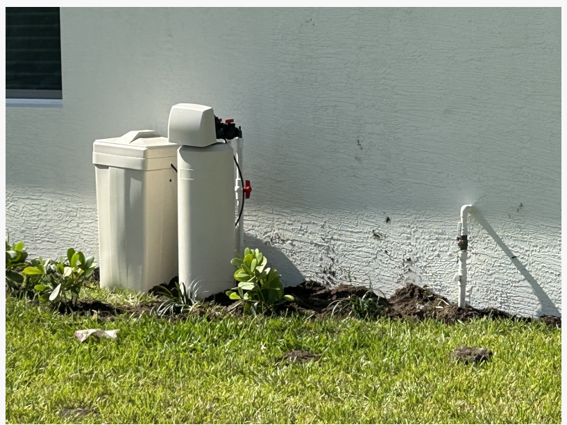
installation of softener in Port St Lucie
