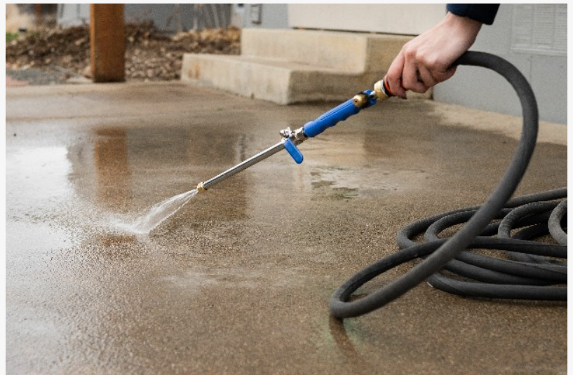
concrete cleaning VIC
