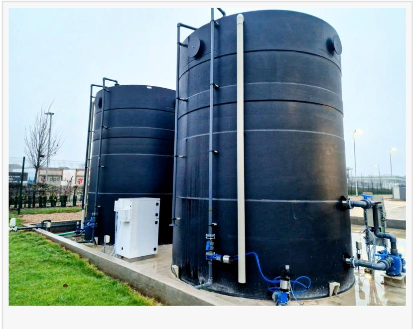
The newly installed bulk storage tanks each boasts an impressive operating capacity of 48,000 litres, with an additional 10% ullage allowance. This expansive capacity permits the [Ogden Water Ltd.](#) treatment plant to handle current and forecast quantities of effluent produced by the food manufacturer.
