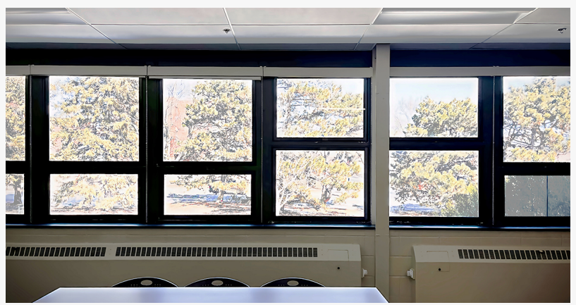
UMN retrofitted fixed and operable windows showcasing INOVUES' non-invasive Insulating Glass Retrofit (IGR) system. Photo by W. L. Hall, the installer.
