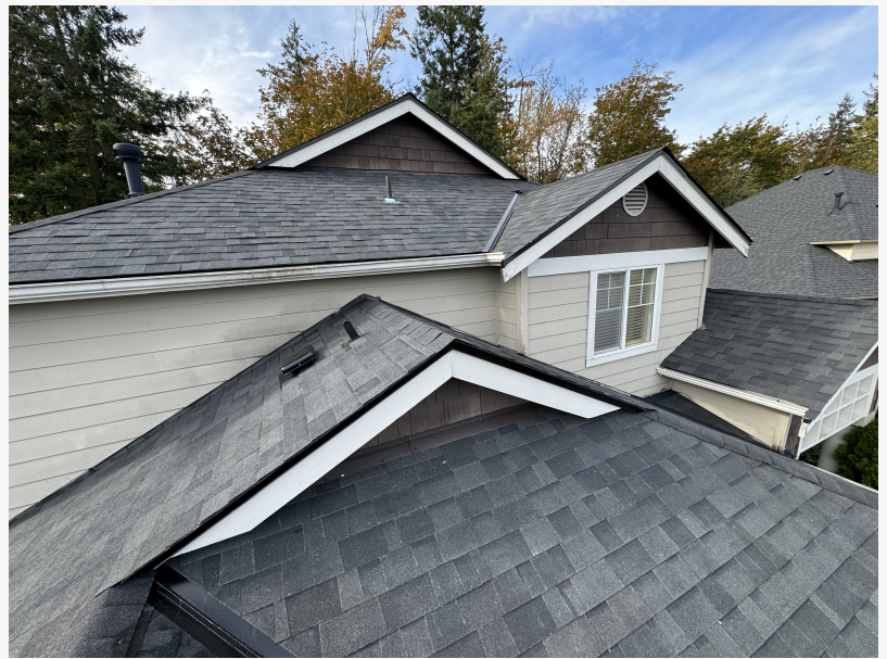
Lake Construction & Roofing, Roof Replacement.
