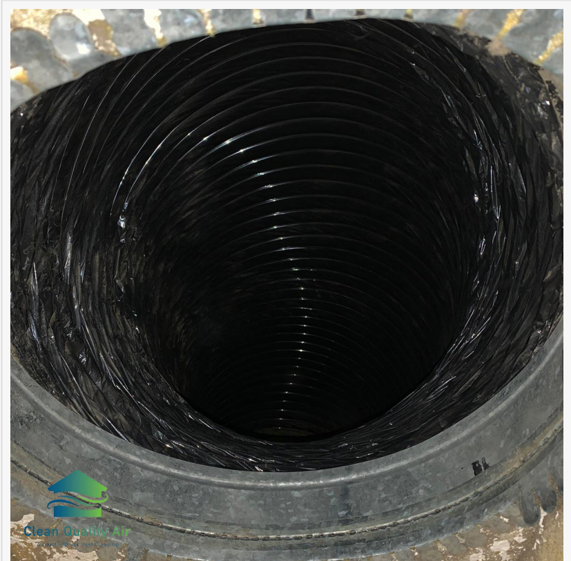
Air Duct Cleaning Services
