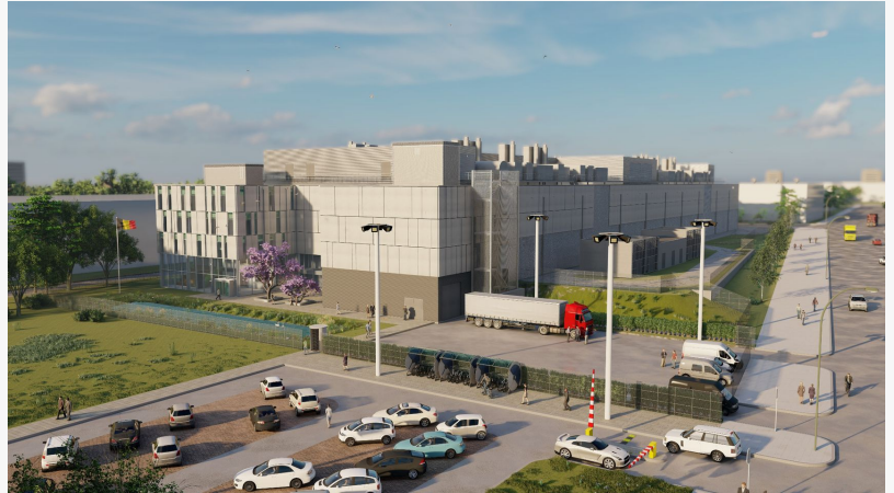
The new 32 MW KEVLINX BRU01 data centre in Brussels will be cloud and hyperscale ready. It is scheduled for completion in 2025
