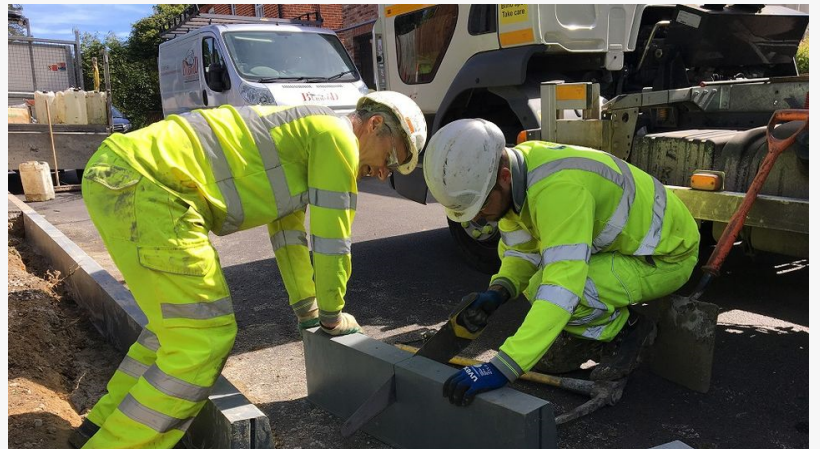
Installation of Durakerb unit
